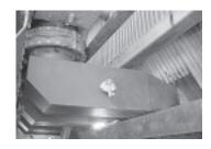
a function of the boiler's combustion hardware, particularly the quality of overfire air (OFA) delivery.
