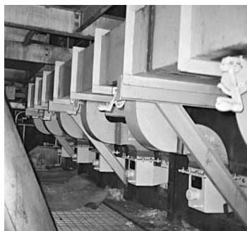
Five of six Jansen OFA nozzles are shown on the front wall of this biomass boiler, including supply windbox, ducting, and supports.
