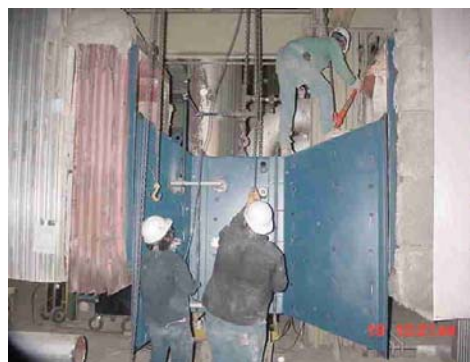
Figure No. 12 Secondary Air Venturi
